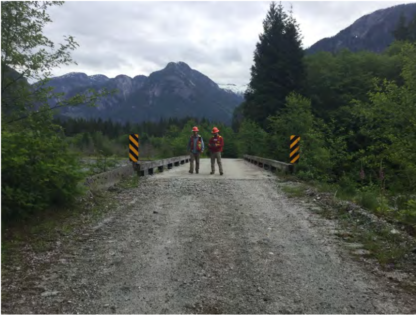
Approach from Right Bank when facing downstream
