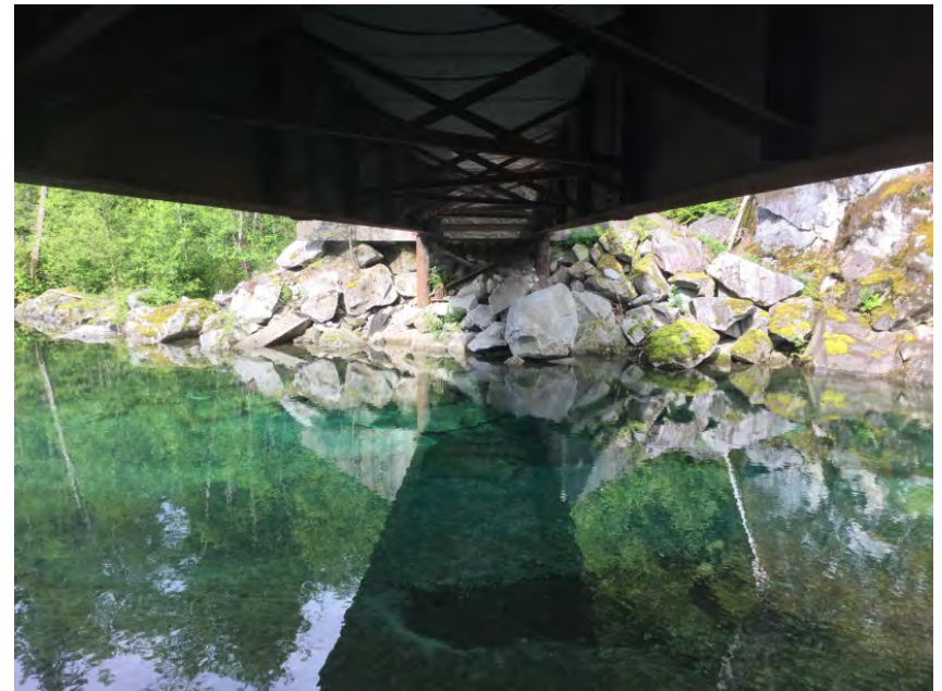
Right Bank Abutment when facing downstream
